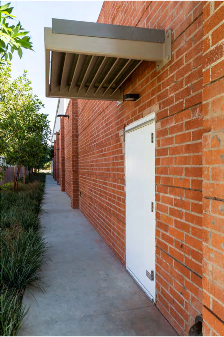
15. Exterior, north façade, view east
