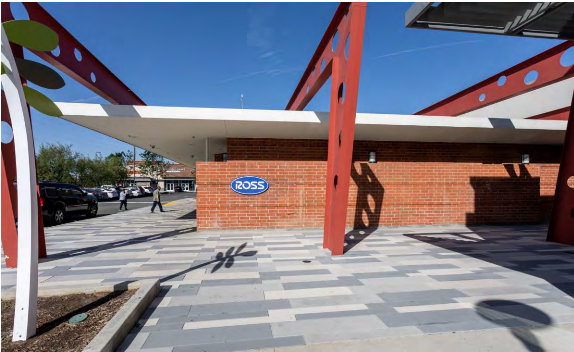
7. Exterior, south façade, view north
