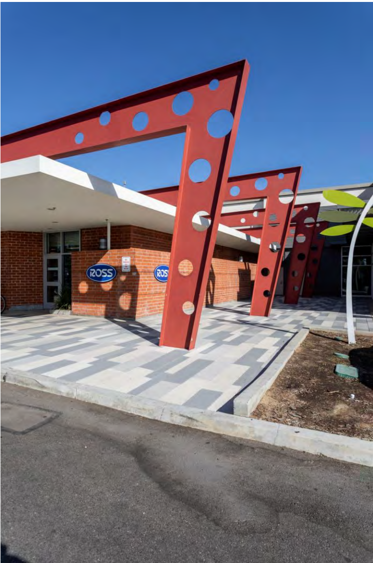
5. Exterior, south façade and “Swiss cheese” steel I-beams, view northeast
