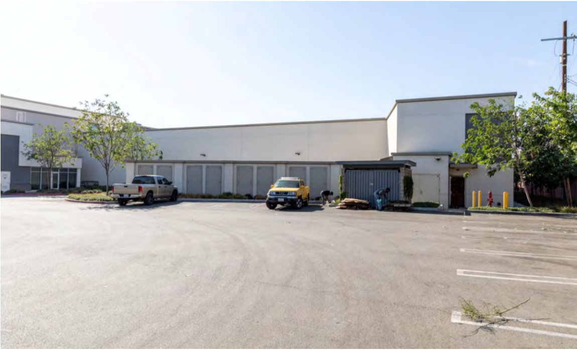
16. Exterior, east façade (addition), view west
