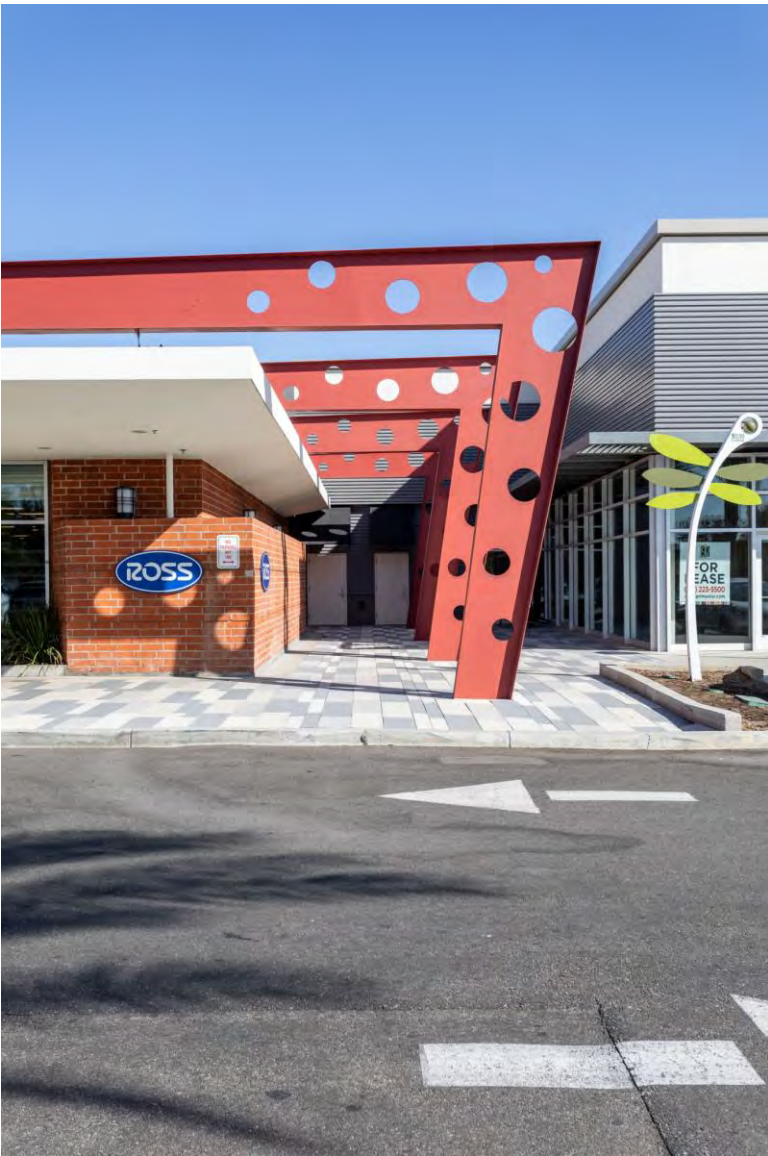
4. Exterior, "Swiss cheese" steel I-beams, view east
