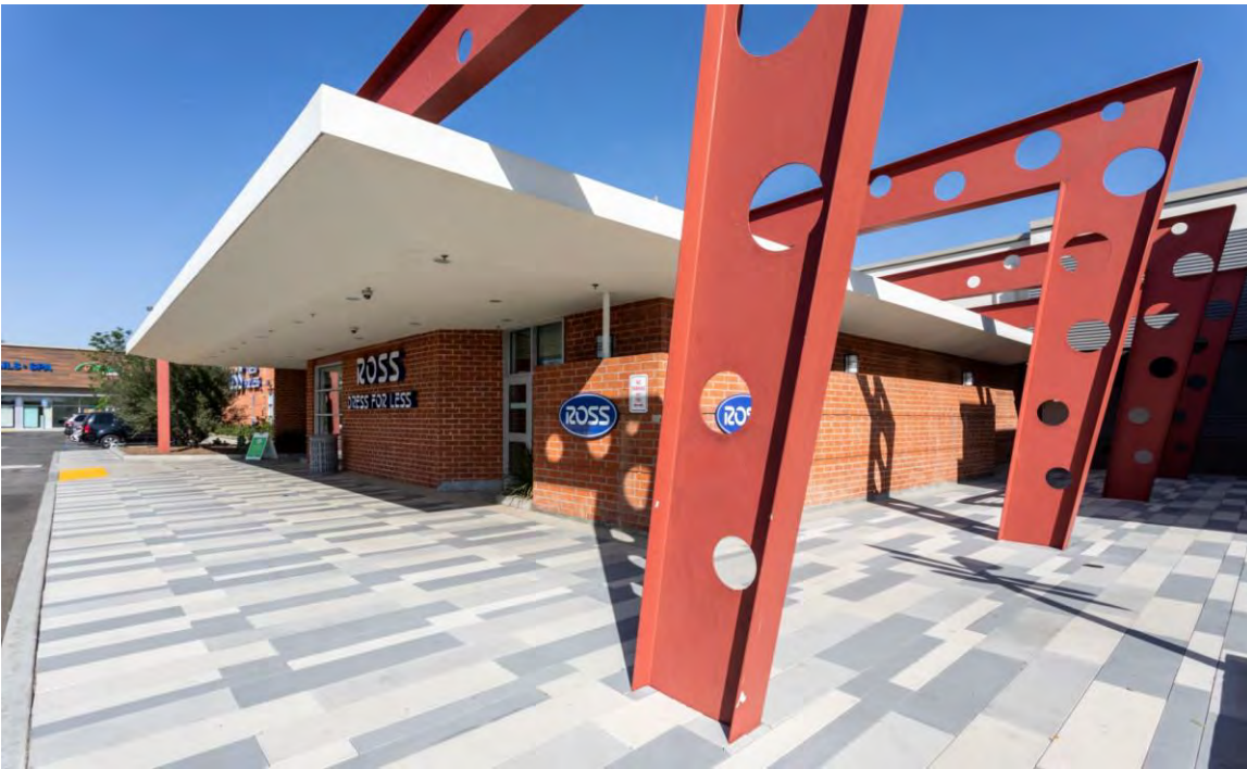
6. Exterior, west and east façades, view northeast
