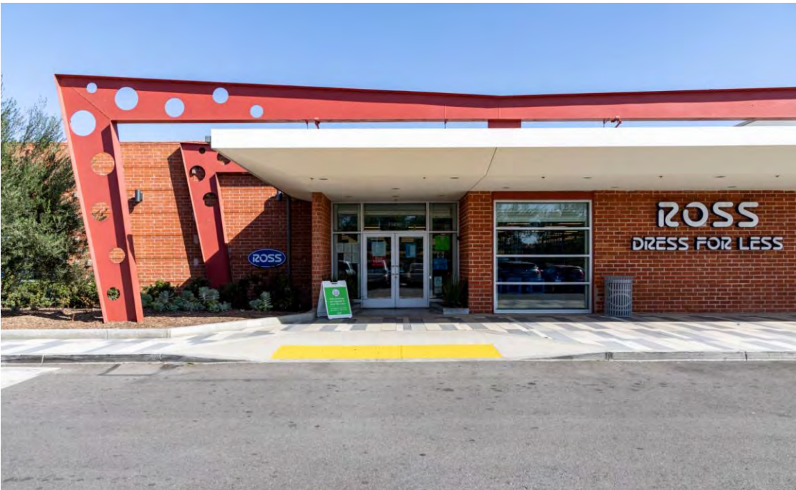
10. Exterior, west façade, primary entrance, view east
