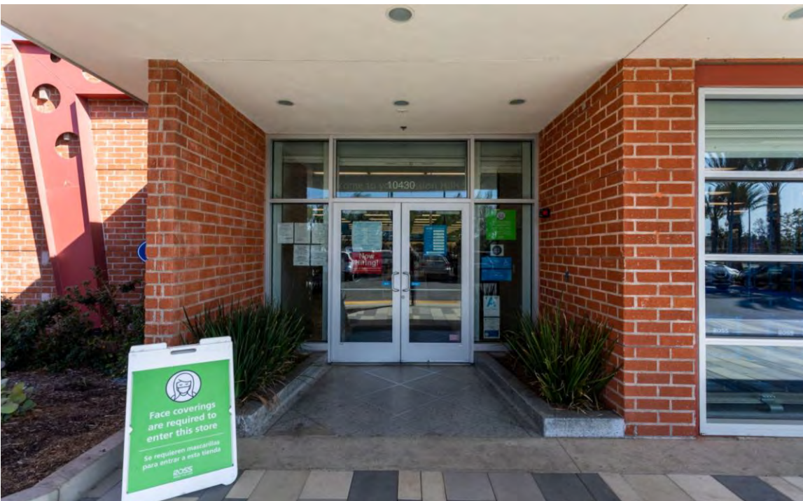
9. Exterior, west façade, primary entrance, view east
