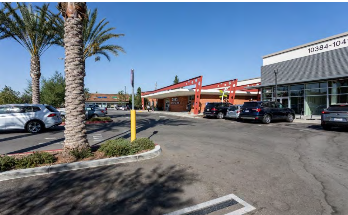
2. Exterior, west and south façades, view northeast
