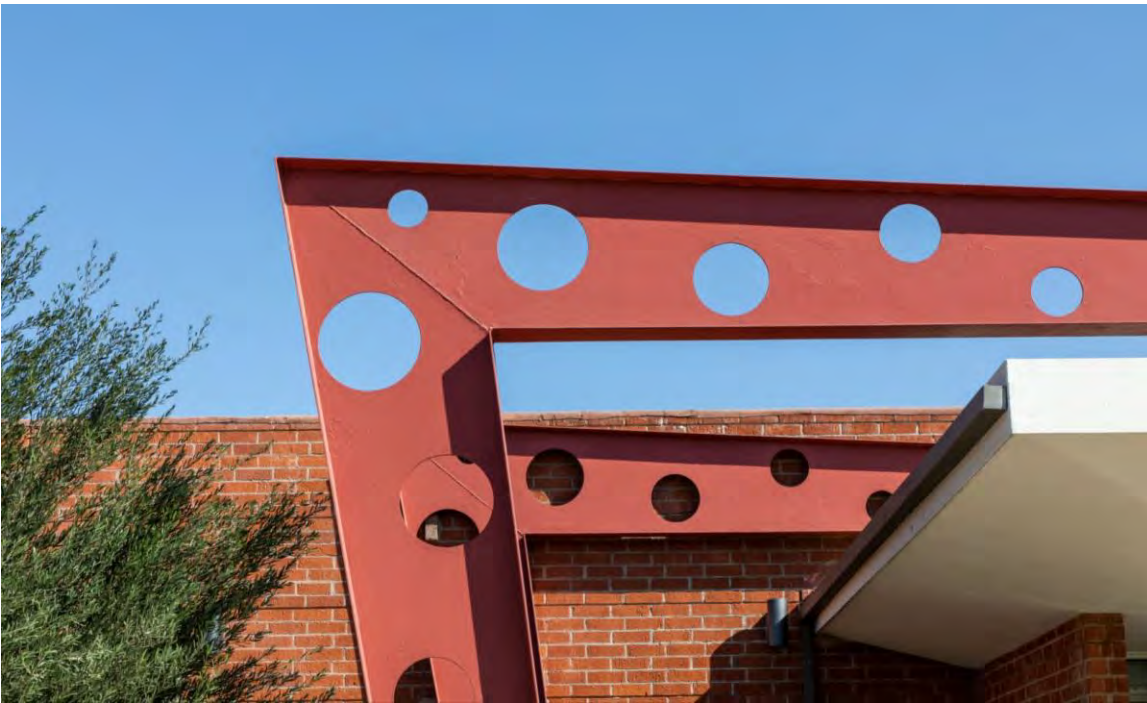
11. Exterior, west façade, "Swiss cheese" I-beams, view east
